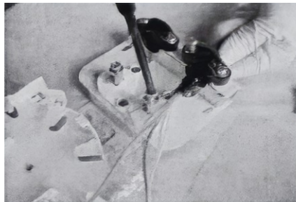
Tighten the strength member clamp
