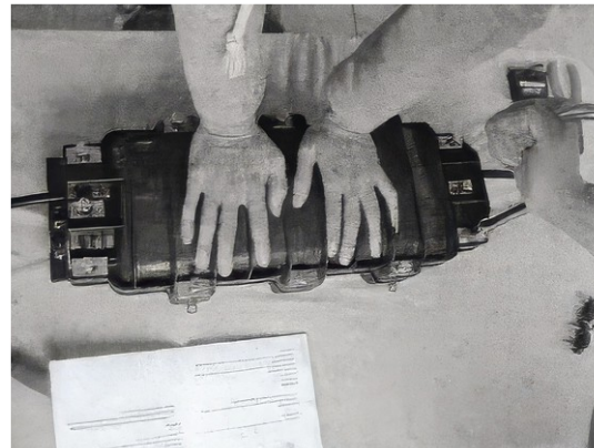
Tighten the fastening bolts
